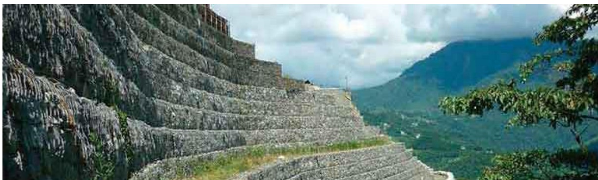
Figura 4.3 Terramesh® System
